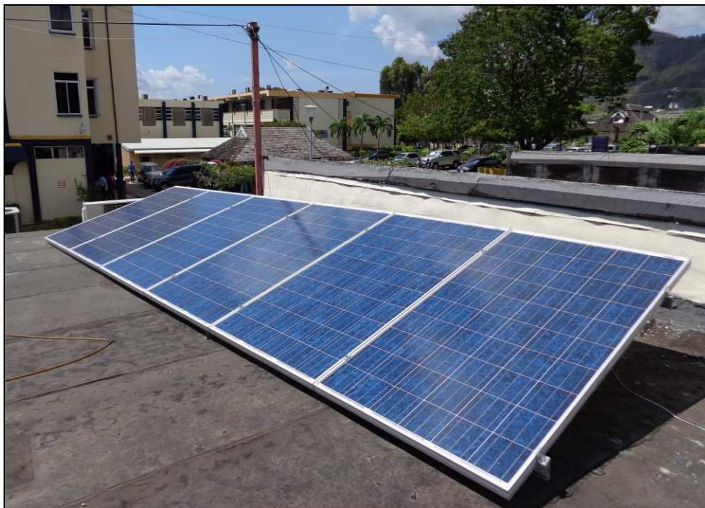
PICTURE 8 – SOLAR INSTALLATION ON THE ROOF OF A TERTIARY INSTITUTION
