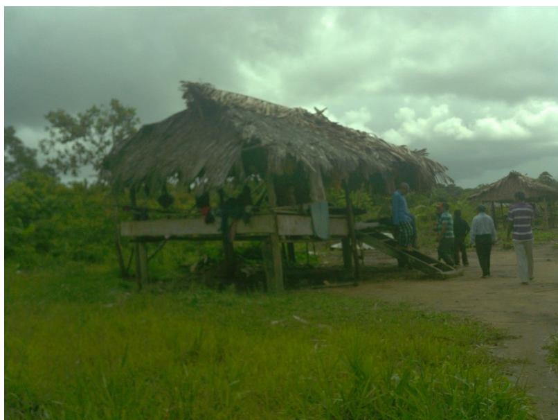
Figure 2: Typical dwelling Powaikoru, June 2014
