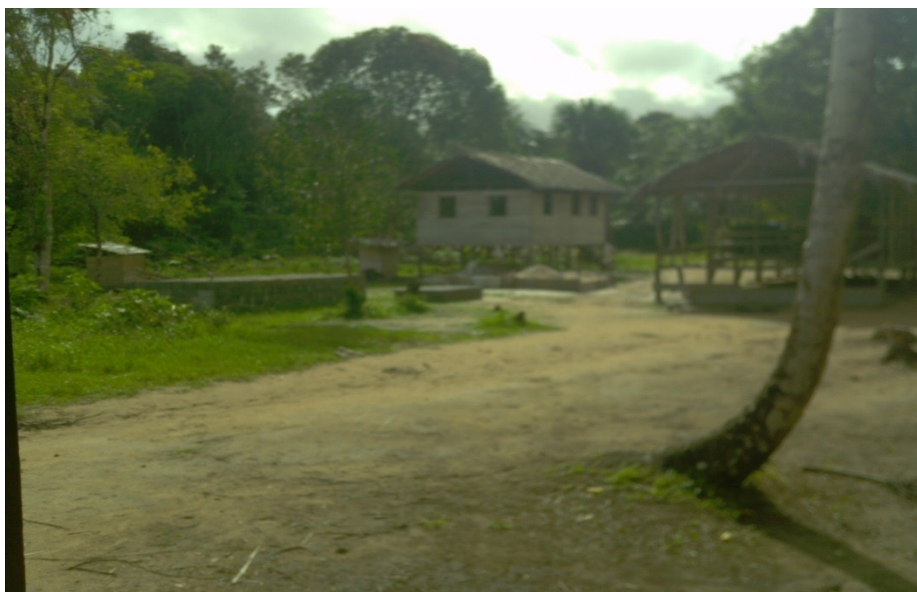
Figure 6: Guest House and Church under construction (foreground) Powaikoru, June 2014
